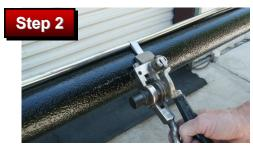
Position the tubing tracer on the pipe wall using tie wire or banding.
