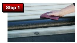
Remove dirt and excessive rust scale from the process pipe using rags or wire brushes.
