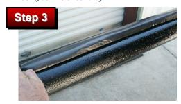
Place a 4 ft. section of Quick Trace over the tracer. Cut bag at both ends.
