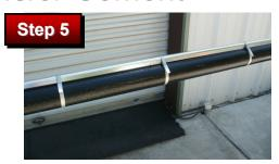
Complete installation by applying three 1/2" wide stainless steel bands for each 4 ft. section of tracing. Measure 18" out in both directions from the center band and secure.
