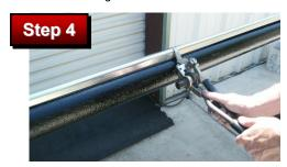
Place the 4 ft. metal channel over the Quick Trace. Attach band at midpoint and tighten.
