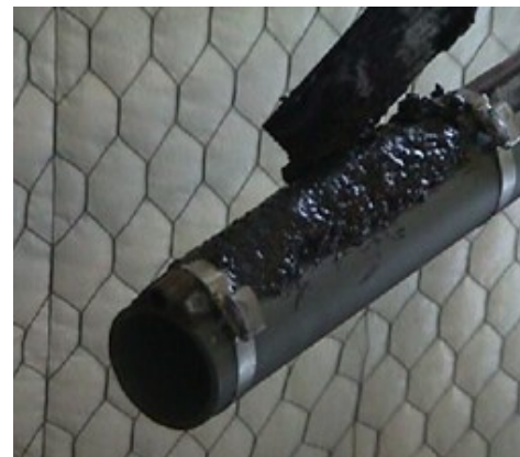
Typical hand trowel application
